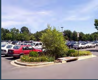
Parking Lot Bioretention
