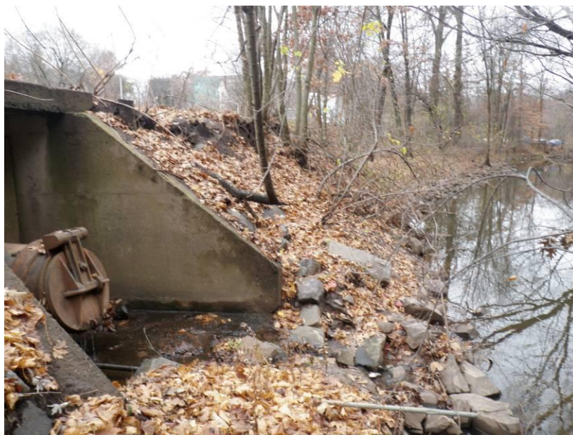
NBP-16: Poor overall condition, with little connectivity to the floodplain, modified bank habitat, and numerous outfalls
