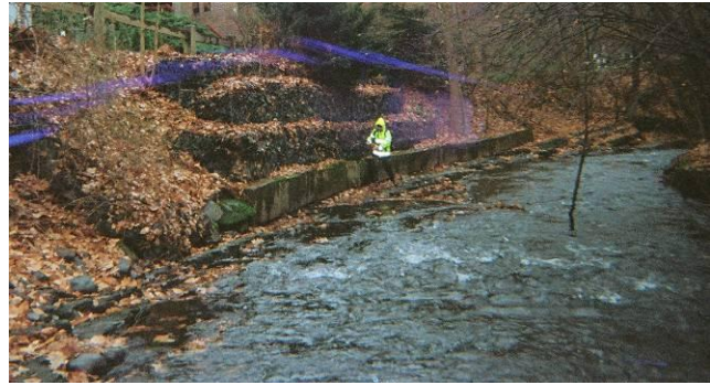
WBS-11: Steep bank reinforced with gabions.
