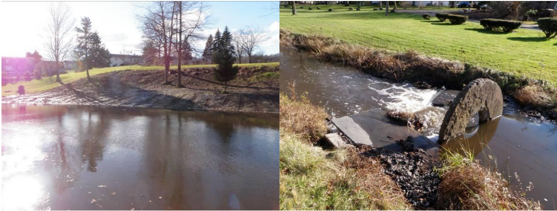
WBS-04: Bank and channel modification and evidence of recent pond dredging.
